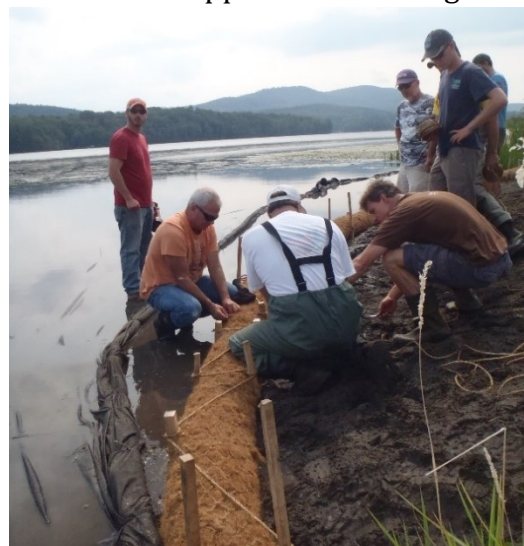
VT Agency of Natural Resources staff get trained in bioengineering methods in 2015 to install fiber coir rolls to stabilize an eroding shore at the Lake Iroquois Fish and Wildlife Access Area in Williston
