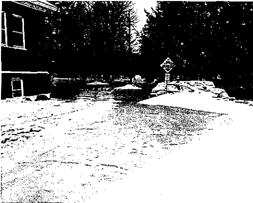
Winter flooding in Johnson, VT
