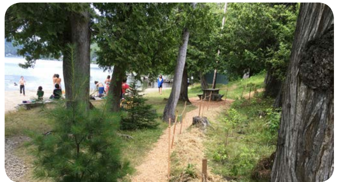
ADA compliant path installed at Brighton State Park.
