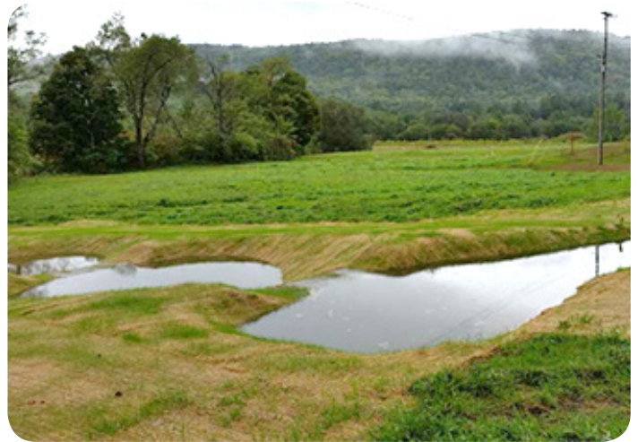
A bioretention system captures runoff from Morey Road in Hyde Park. This project was completed by the Lamoille County Conservation District with Ecosystem Restoration Grant funds.
