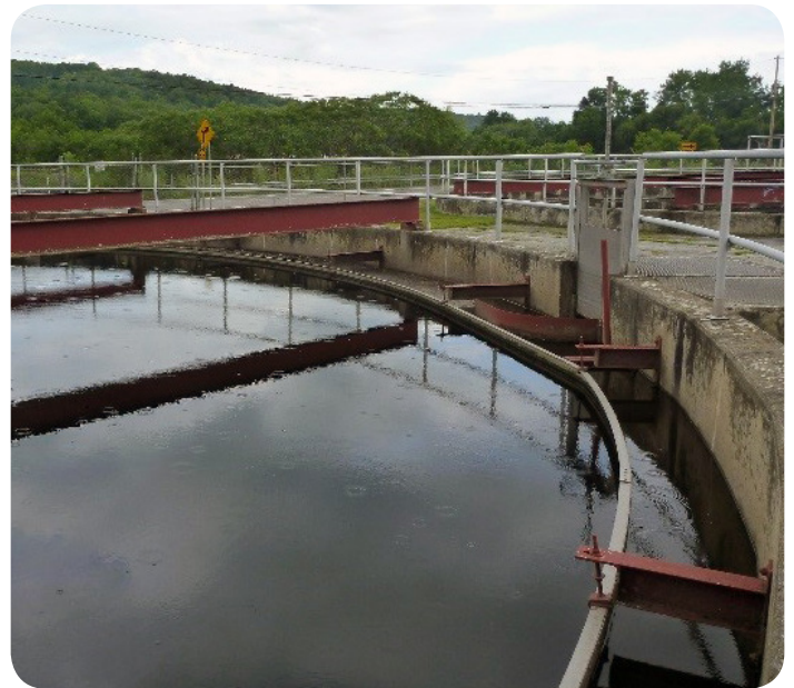
At the Montpelier facility, secondary clarifiers provide a final settling area for material from the aeration basin. Effluent flows over the secondary clarifier weirs to be disinfected and is then safe to be discharged to the Winooski River.
