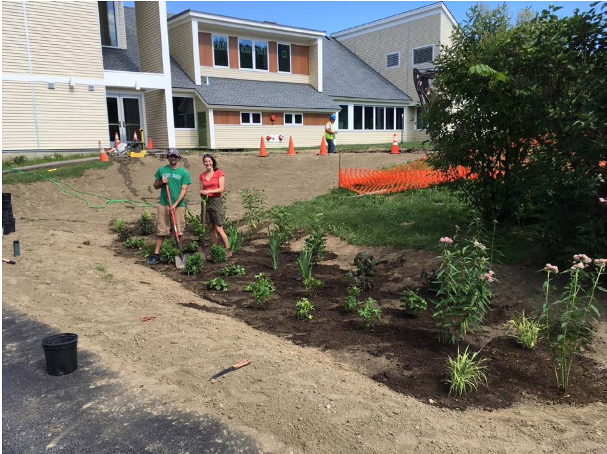
Figure 22. Rain Garden at Warren School
