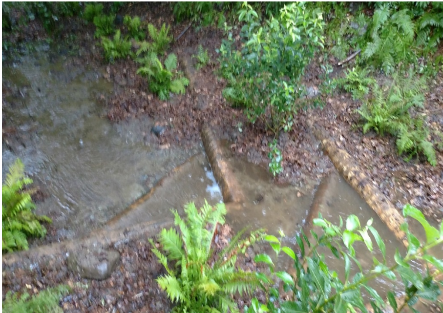
Figure 16. A tributary to Lake Iroquois, where timbers were placed to intercept water flow thereby reducing erosion and trapping sediment.
