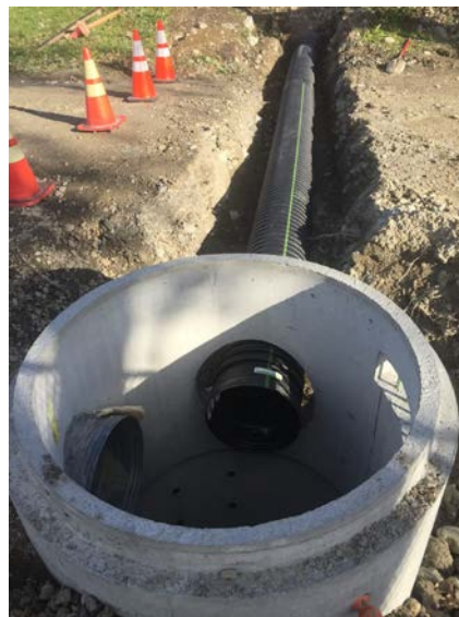
Figures 11 and 12. Stormwater treatment practices installed at Castleton Transfer Station
