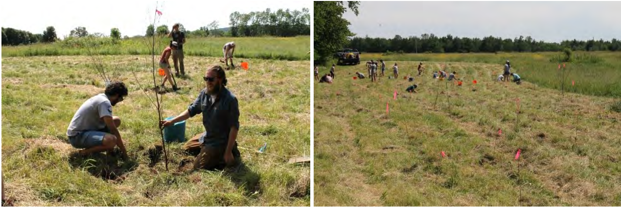
Figure 28. Before (left) and after (right) remediation of gully with bio-engineering near Crooked Creek in Colchester, completed by Fitzgerald Environmental Associates with ANR funding
