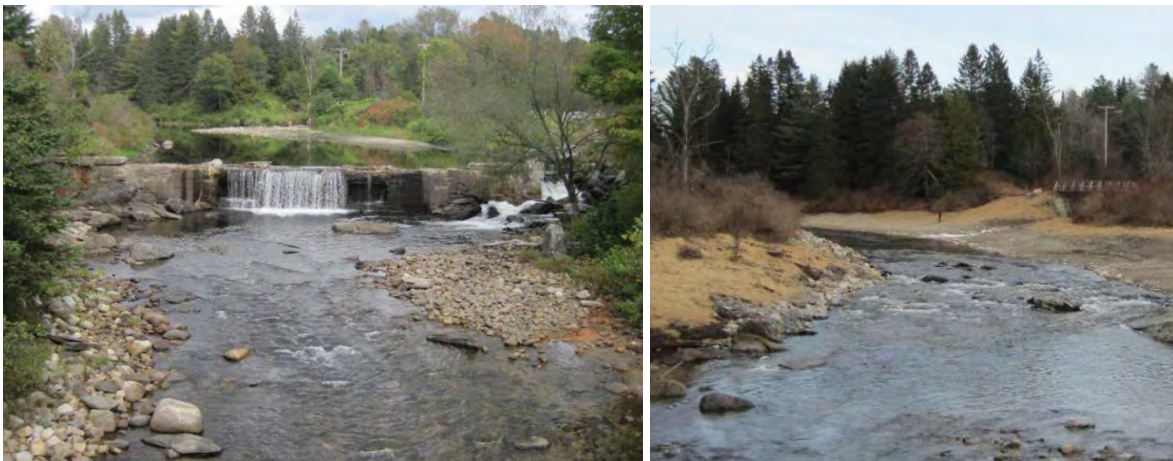
Figure 29. Before (left) and after (right) removal of dam on the Passumpsic River in East Burke, completed by Connecticut River Conservancy with ANR funding
