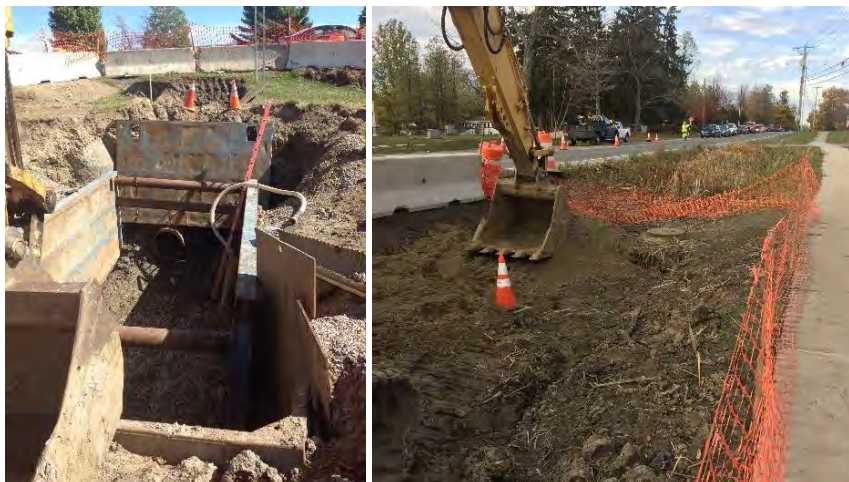
Figure 25. Construction of sewer replacement under Vermont Route 2A in Williston completed by Town of Williston with financing from the Vermont and EPA Clean Water State Revolving Fund (CWSRF)
