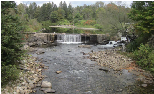
Before removal of the East Burke Dam on the East Branch of the Passumpsic River
