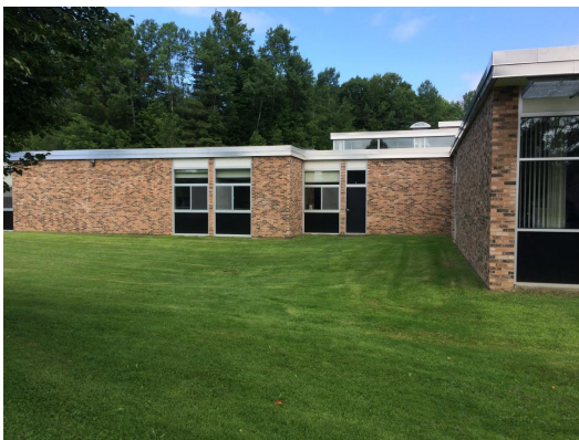
Area outside classroom before bioretention was installed
