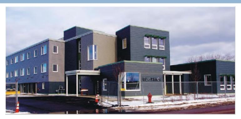
Only 127,651 kBTU/yr at 2°F for 27,690 sqft floor area A 20 kW PV rooftop array produces 67,085 kBTU/yr
