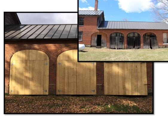
Replicated severely deteriorated doors and hinges
