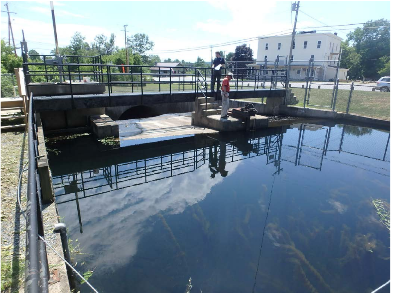
Lake Bomoseen Dam, minor repairs
