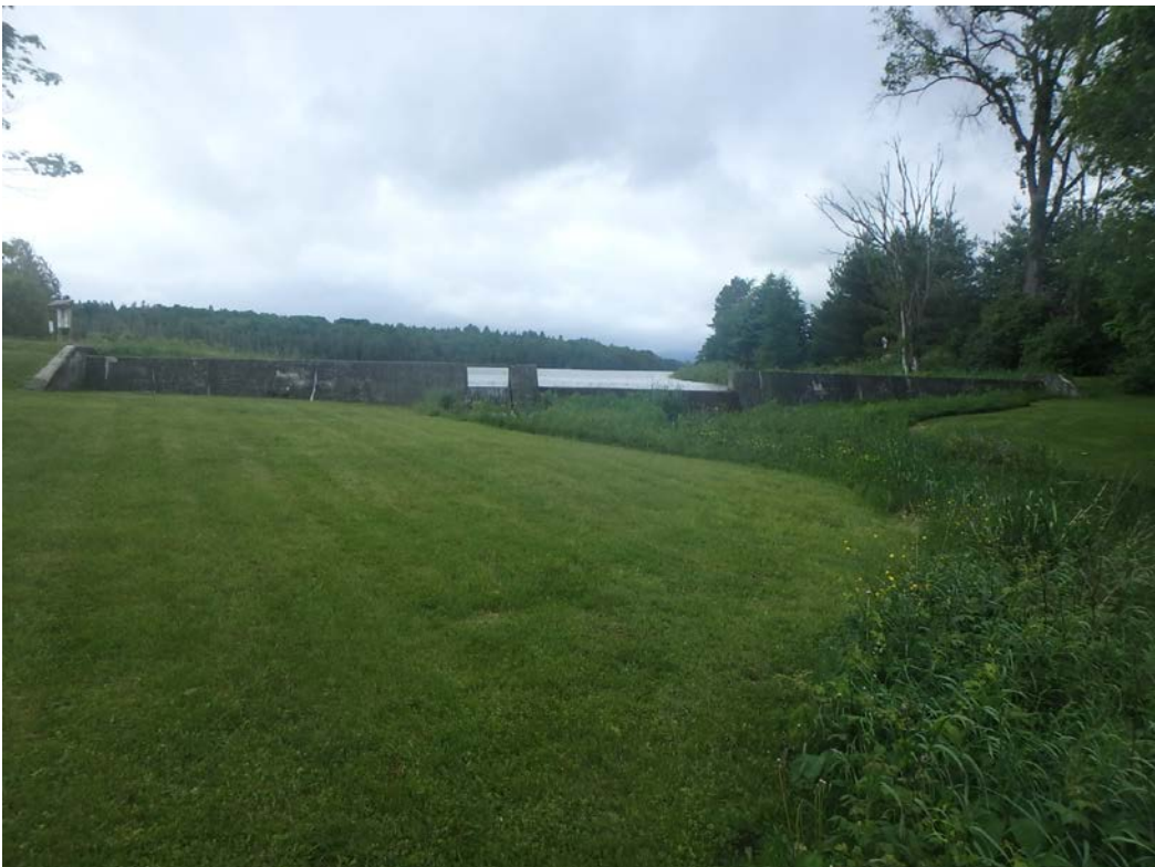
Little Hosmer Dam, assessment, design, rehabilitation construction
