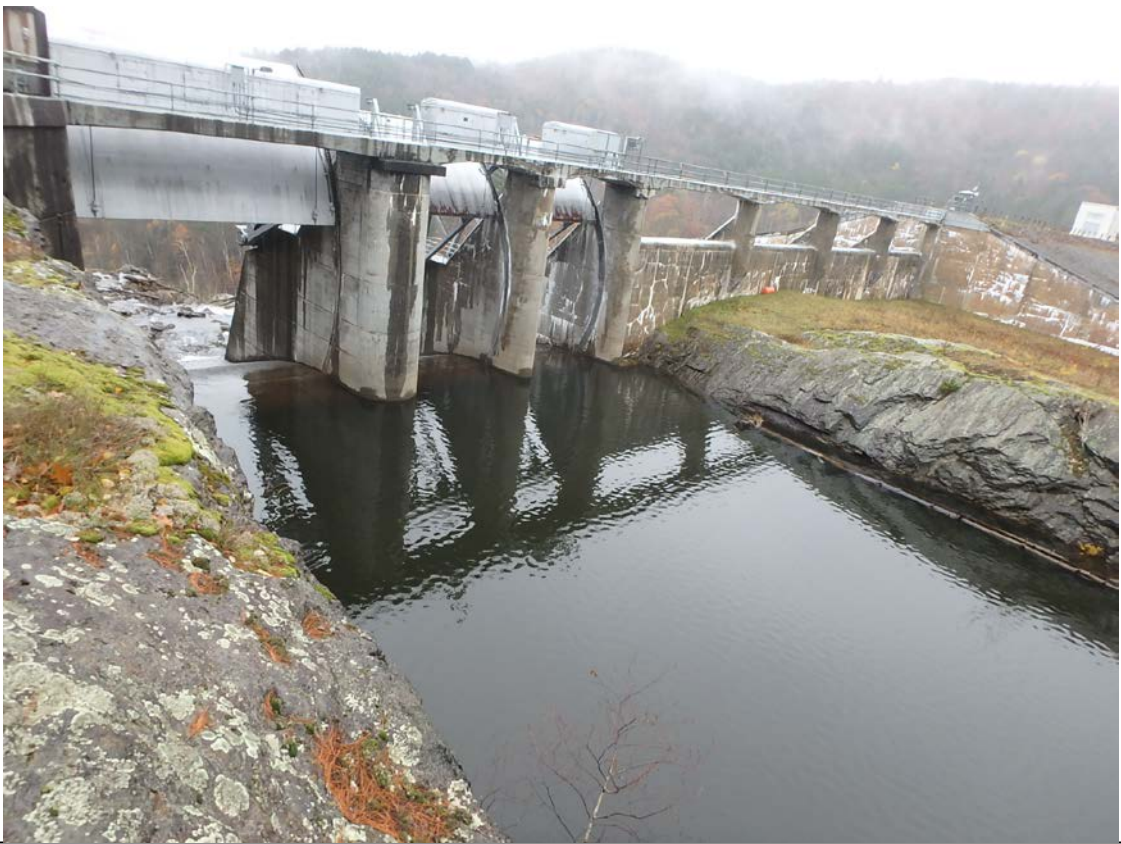
Waterbury Dam Spillway Replacement, Risk Assessment, $215k from previous years. The approach channel in need of a new boat barrier can be seen.
