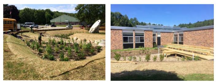
Figure 24. Before (left) and after (right) installation of road erosion remediation along Long Hill Road, Concord by the Town of Concord in partnership with Northeastern Vermont Development Association through the Municipal Roads Grants-in-Aid Program
