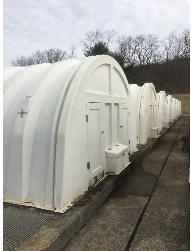
Figure 31. Replacement of rotating biological contactors (RBC) for wastewater treatment, completed by the Town of Bennington with financing from the Clean Water State Revolving Fund (CWSRF)
