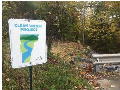
Gully erosion remediation at Pouliot Avenue, Barre Town , completed by Friends of the Winooski River
