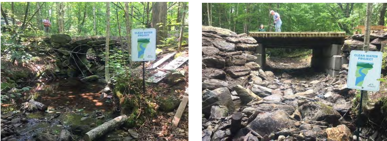
Figure 35. Before (left) and after (right) replacement of a deteriorating, 30-year old culvert with a bridge on Boulley Brook in Johnson completed by Vermont Department of Forests, Parks and Recreation with funding from a DEC Clean Water Initiative Program grant (clean water project sign posted during construction)
