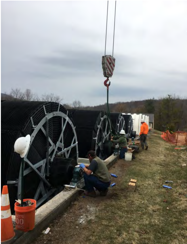
Figure 31. Replacement of rotating biological contactors (RBC) for wastewater treatment, completed by the Town of Bennington with financing from the Clean Water State Revolving Fund (CWSRF)
