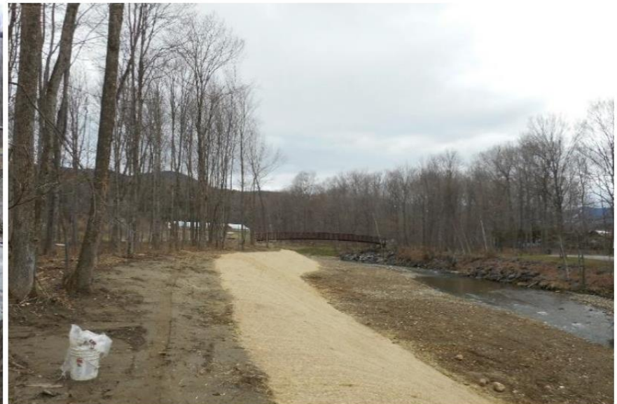
Figure 24. Before (left) and after (right) relocation of 1,100 feet of Stowe's Recreation Path outside of fluvial erosion hazard zone and restoration and planting of 2 acres of floodplain, completed by Town of Stowe
