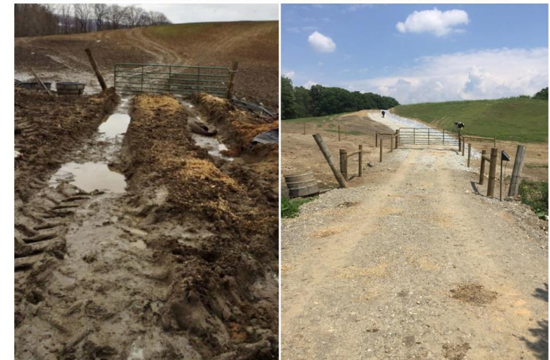
Figure 21. Before (left) and after (right) installation of livestock exclusion fencing and improved laneway and water crossing, completed by Poultney Mettewee Conservation District with ANR funding
