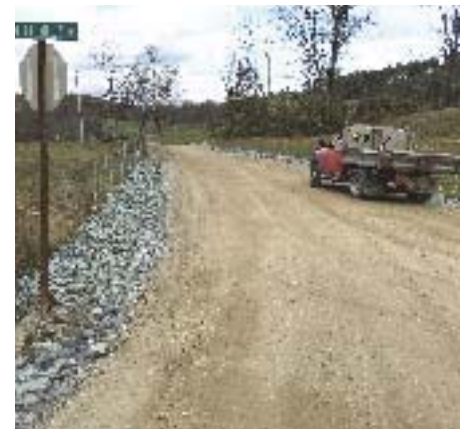
Before (left) and after (right) installation of a stone-lined ditch along Finel Hollow, Highland Gray, and Watkins Hill Roads in Poultney, completed by the Town of Poultney with VTrans funding
