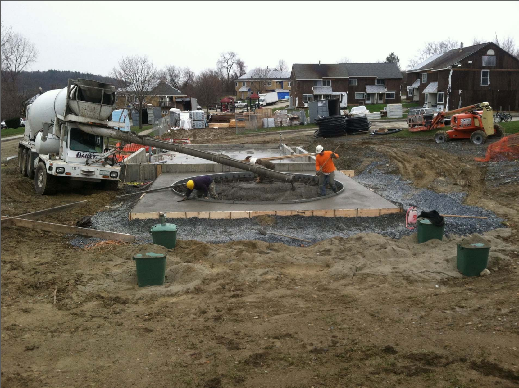
Foundation work underway on the central biomass heating system building.
