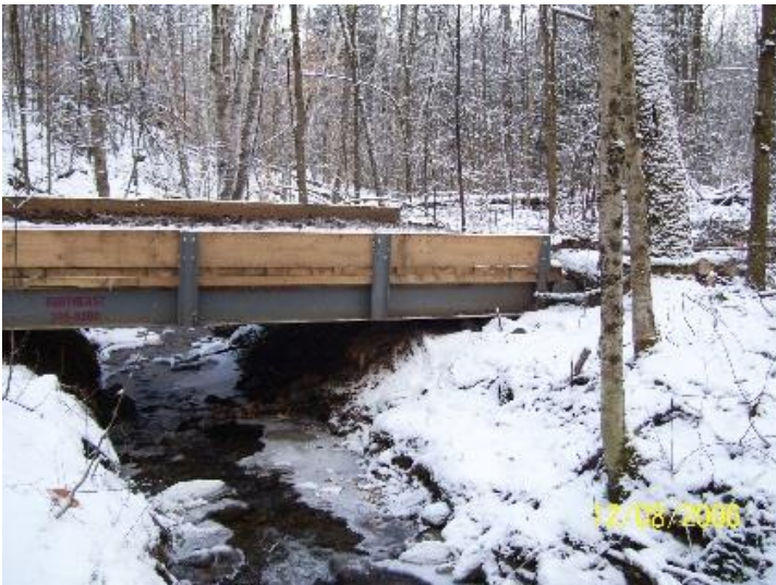
Wood over steel skidder bridges
