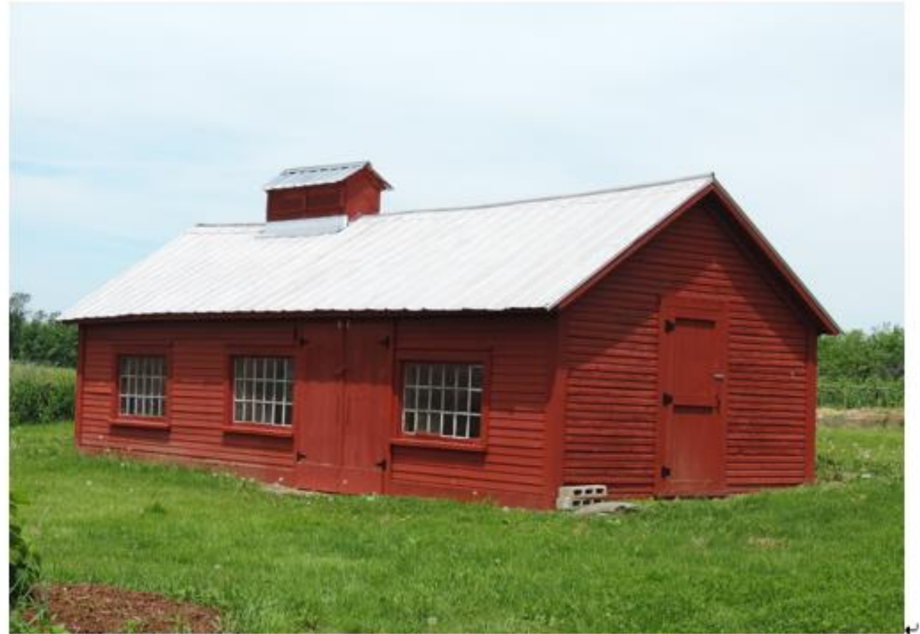
Pearl House Farm, Grand Isle $11,650 to restore a former sugarhouse
