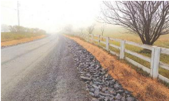
Ditching, St. Johnsbury
