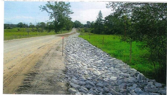
Fairfield, VT After
