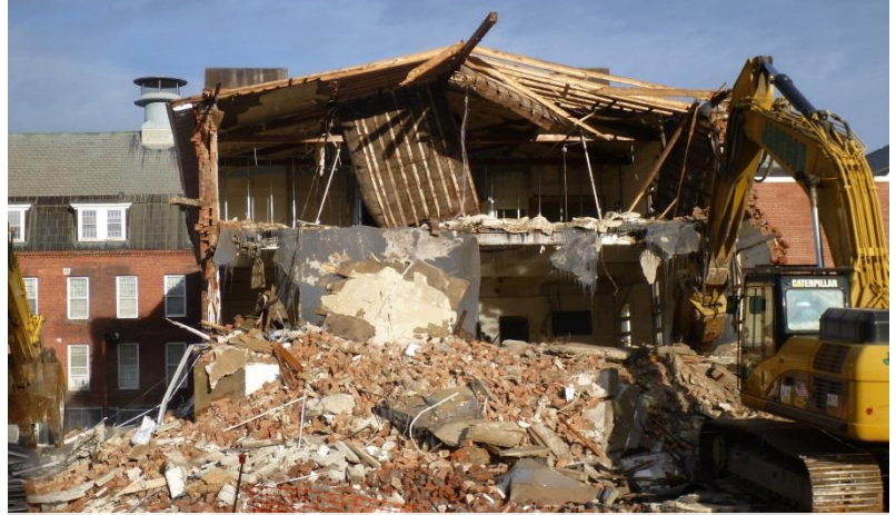
Construction and demolition project site at a former State office complex in Waterbury, VT.
