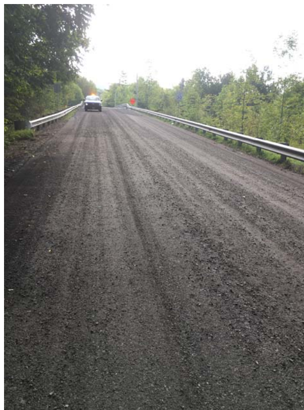
September 2016 installation in Brookfield
