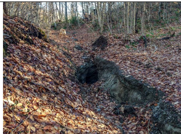
Photo 2 Direction E Date 11/7/2016 Subject: Waterbar destroyed by ATVs above headwall erosion in trail.
