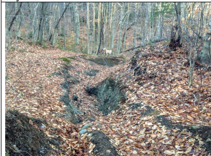
Photo 5 Direction W Date 11/7/2016 Subject: Severe erosion just below a waterbar compromised by ATVs.
