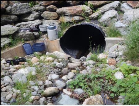
Photograph 2. Automated sampler at Access Road culvert inlet, upstream from LS-A9 vegetated buffer area (VHB, 07/08/16)
