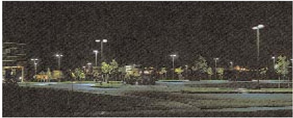
Cut-off lamps such as these will eliminate glare in parking areas. Source: Outdoor Lighting Manual for Vermont Municipalities.
