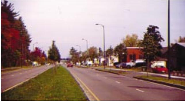
A median provides greater control over left turn movements, channeling them to intersections. This technique keeps traffic flowing and provides an aesthetic benefit.
