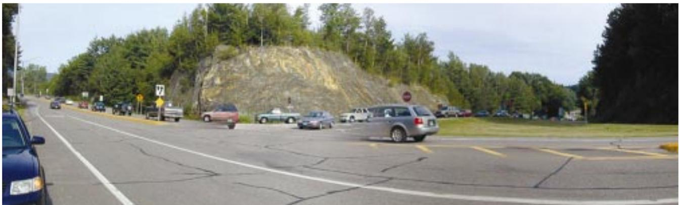
Rte. 100 in Waterbury intersecting I-89 Exit 10 is an arterial road that is sometimes overwhelmed by increased traffic. In a short exit ramp, without additional capacity to accommodate waiting vehicles, cars can back up to the travel lane of the interstate, posing a safety hazard.
