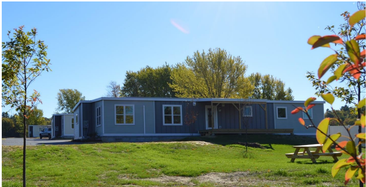
McKnight Lane is a 14-unit net-zero affordable housing development a mile from downtown Vergennes.
