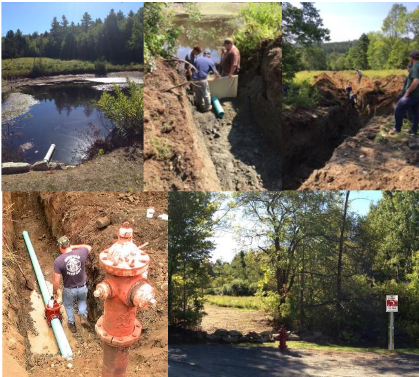
New "wet" Hydrant in Windham
