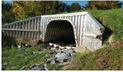
Stream culvert replacement completed by the Town of Cambridge (see Figure 29)
