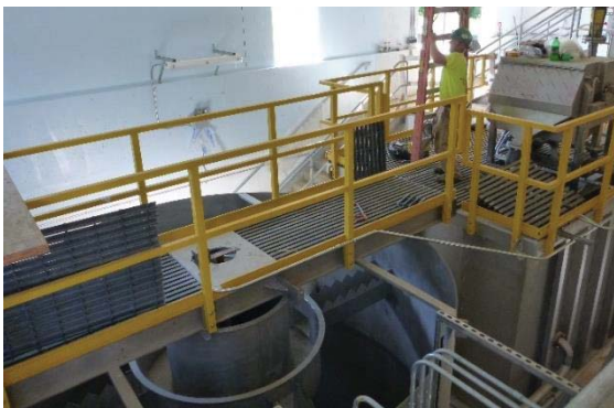
Figure 30. Construction of the Waterbury WWTF phosphorus removal upgrade, completed in 2016
