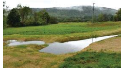
Bioretention system on Morey Road, Hyde Park completed by Lamoille County Conservation District (see Figure 27)
