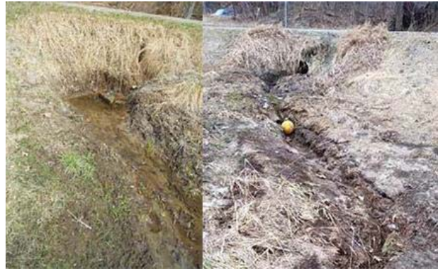
Figure 27. Before (top) and after (bottom) installation of bioretention system on Morey Road in Hyde Park, completed by Lamoille County Conservation District
