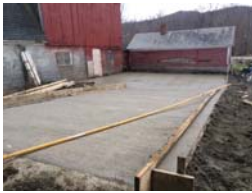
Stabilized concrete walkway completed by Poultney Mettowee Conservation District (see Figure 23)
