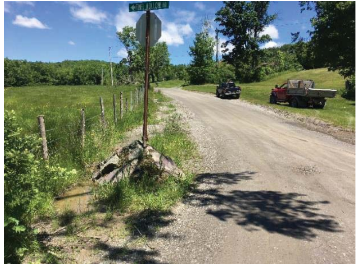
Figure 28. Before (left) and after (right) installation of a stone-lined ditch along Finel Hollow, Highland Gray, and Watkins Hill Roads in Poultney, completed by the Town of Poultney.
