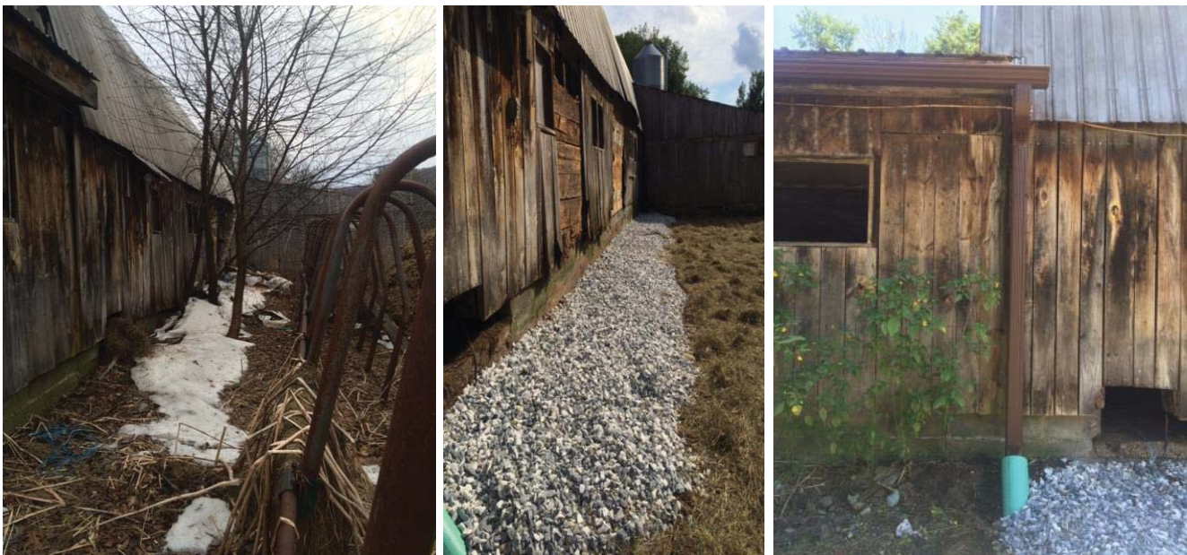
Figure 22. Before (left) and after (middle and right) installation of barnyard roof runoff diversion practices, completed by Poultney Mettowee Conservation District with ANR funding
