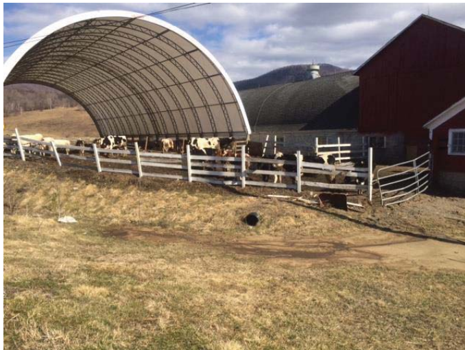
Figure 23. Before (top) and after (below) installation of concrete walkway to stabilize pathway from hoop barn to milking barn, completed by Poultney Mettowee Conservation District with ANR funding
