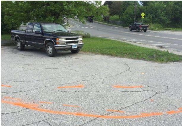
Figure 26. Before (top) and after (bottom) installation of bioretention system on Center Street in Northfield, completed by Central Vermont Regional Planning Commission
