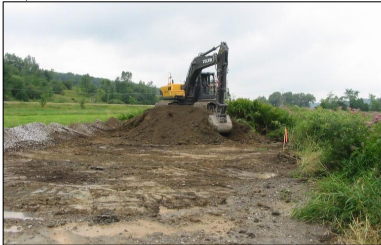
3/3/2017 Removal of elevated railroad embankment
