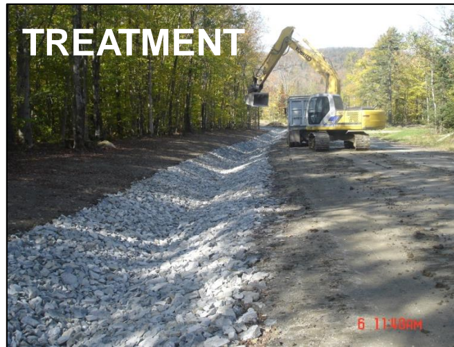
Ditch stabilization saves road and reduces erosion
