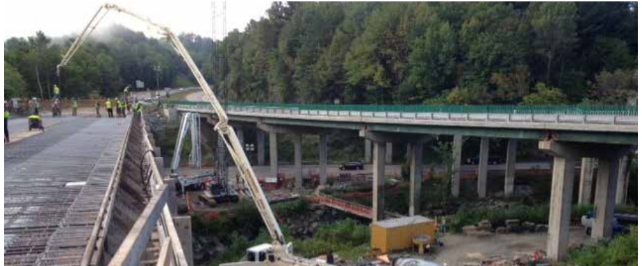
WATERBURY. Construction of I-89, Exit 10 north bound off-ramp bridge.
