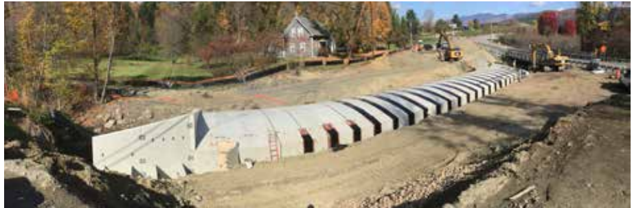
DUXBURY. Construction of new Precast Concrete Rigid Frame culvert on VT 100.
