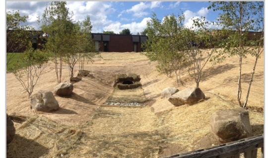
Infiltration gallery at Morrystown Elementary School, a Green Stormwater Infrastructure (GSI) practice installed by the Lamoille County Conservation District
