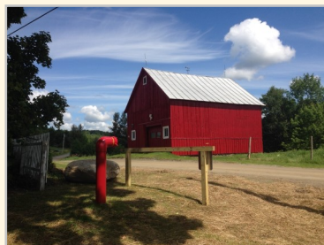
Dry hydrant installed in Enosburg
