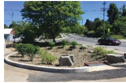
Bioretention system on Center Street, Northfield completed by Central Vermont Regional Planning Commission (see Figure 26)
