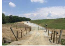
Livestock exclusion fence and improved laneway completed by Poultney Mettowee Conservation District (see Figure 21)
