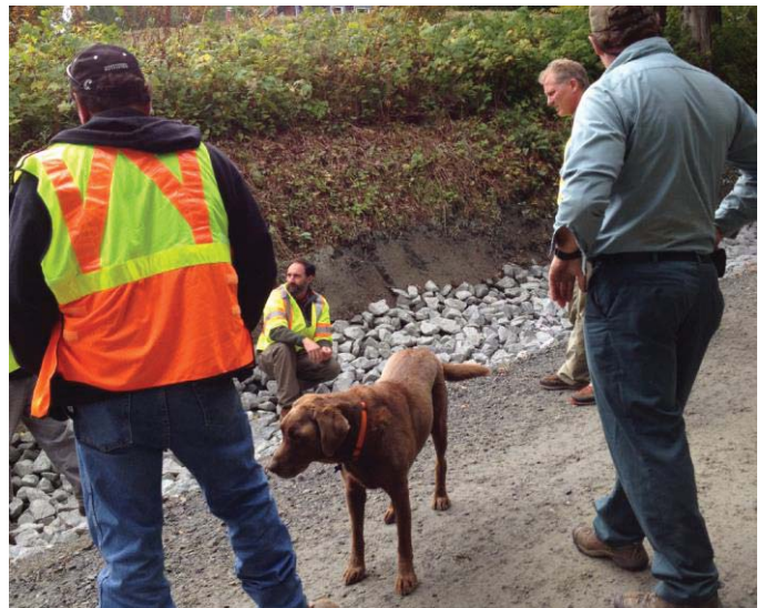
VTrans and DEC staff visiting a stone-lined ditch during a site visit
