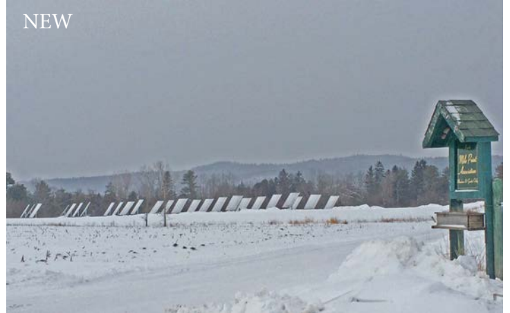
New view from entrance of Mile Point Road; array is size of a football field (150' x 350'); 25 Trackers each the size of two UPS trucks stacked (22' wide x 20' high).
