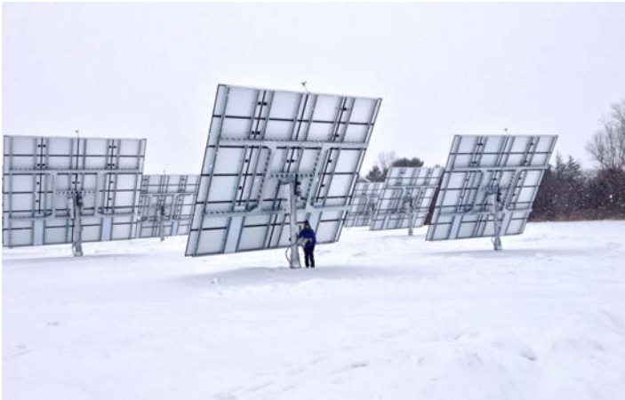
View from Mile Point Road looking south-southwest; note scale compared to person in photo. Hedgerow visible on right.
