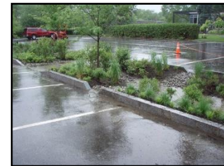
Green infrastructure captures stormwater runoff
