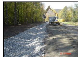
Stabilizing eroding ditch
