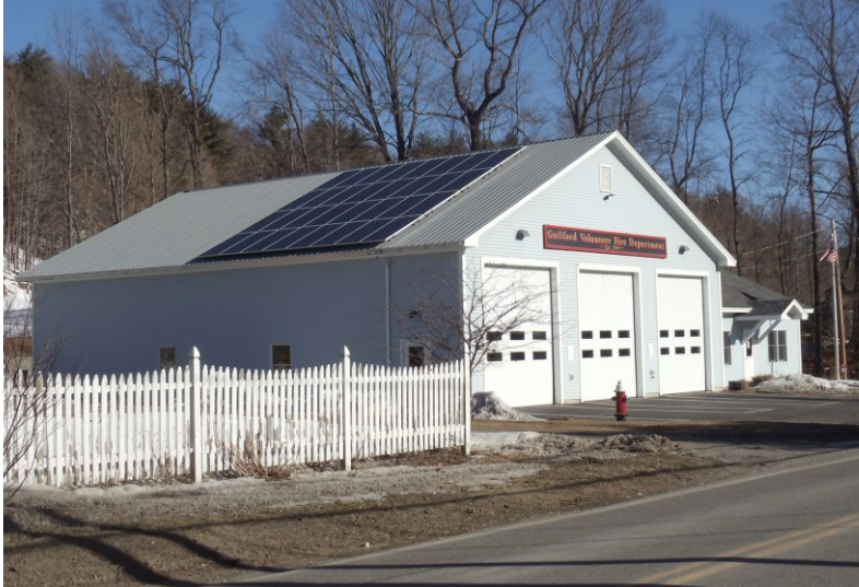
Guilford Fire Department's 10kW system.
