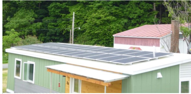
6 kW PV system on a net zero home for the Twin Pines Housing Trust.
