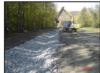
Stabilizing eroding ditch
