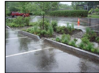
Green infrastructure captures stormwater runoff
