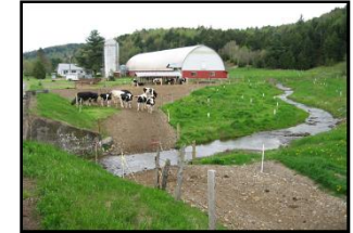
Installation of livestock fencing & buffer
