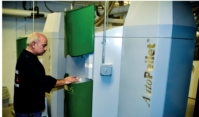
Marc Brown with Burke Town School's new wood pellet boiler.
