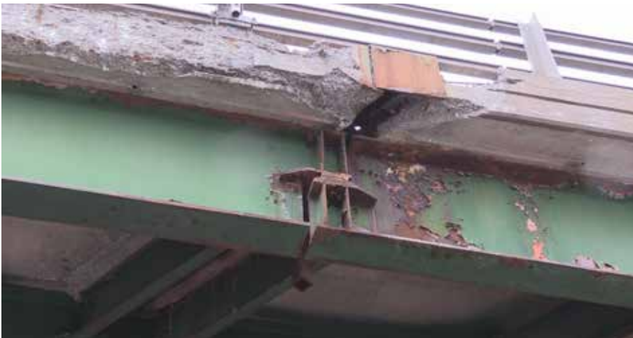
HARTFORD. One of the I-91 bridges.
