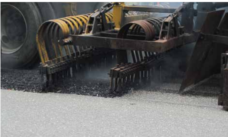
Hot recycled in place pavement.
