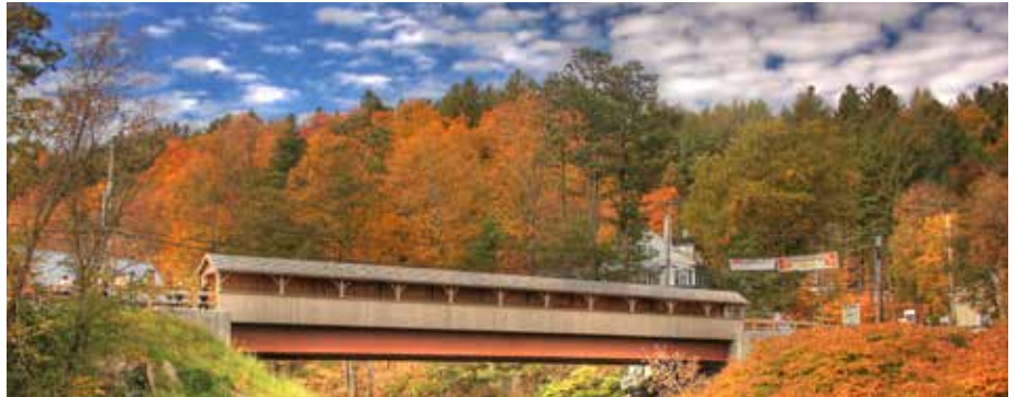
STOWE. Bridge 2, located in the heart of Stowe Village along VT 108, was replaced using innovative construction techniques during a 40 day closure in April and May of 2015.
