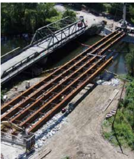
RUTLAND. River Street town highway bridge.
