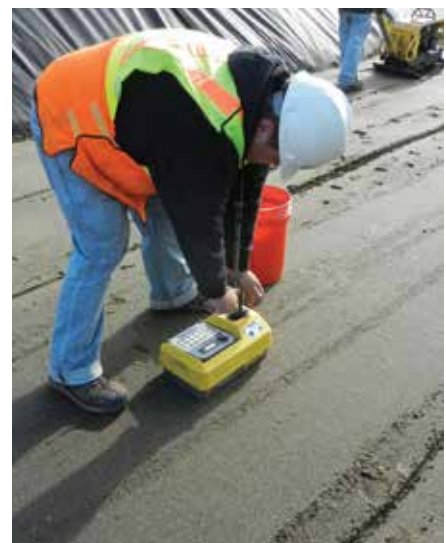
Testing material density.
