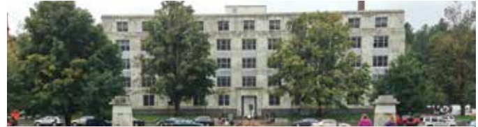
MONTPELIER. DMV main office.
