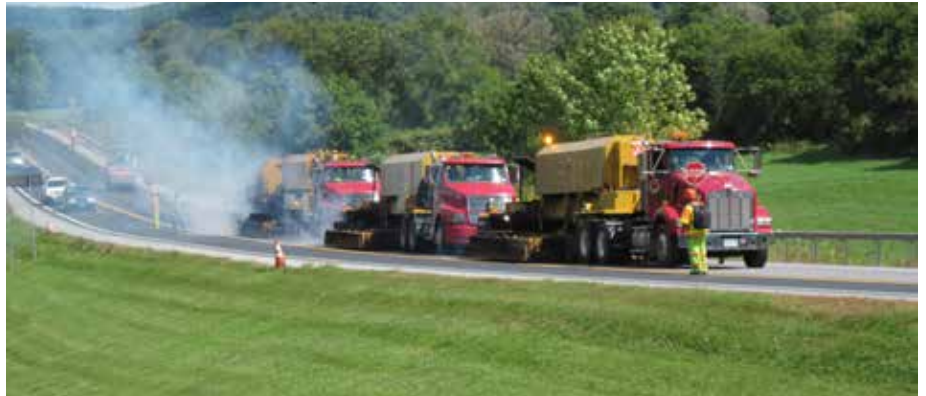
WAITSFIELD / MORETOWN. Paving project.
