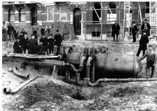
Figure 1 Vacuum-pumping-station in Amsterdam July 1873 (source: Roediger company, published in Lange, 2002). In Amsterdam in 1906 more than 4,500 vacuum toilets were connected to a Lienur-vacuum-system
