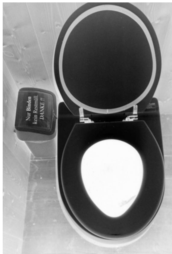
Figure 4: Toilet stool with black removable insert and sealing
