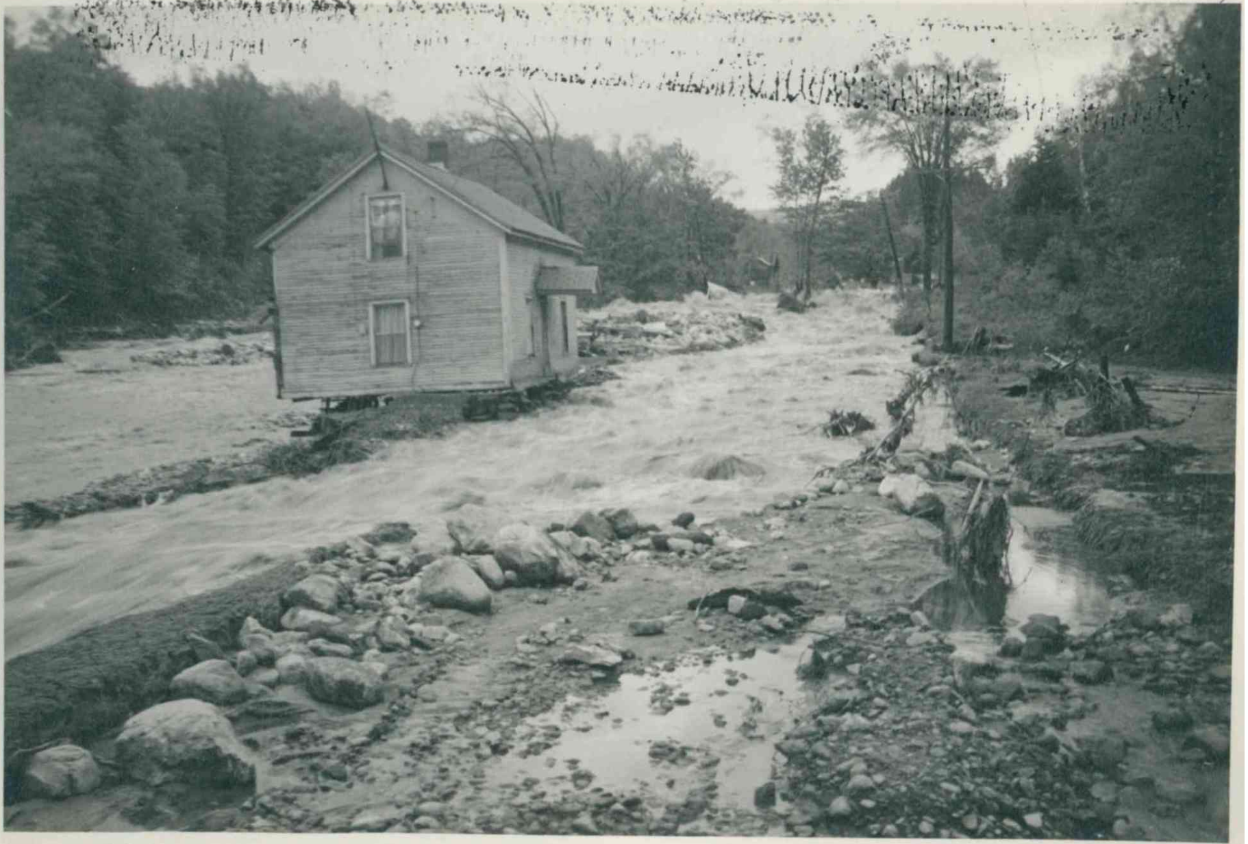
A Chittenden house dragged down stream to sit squarely in the brook
