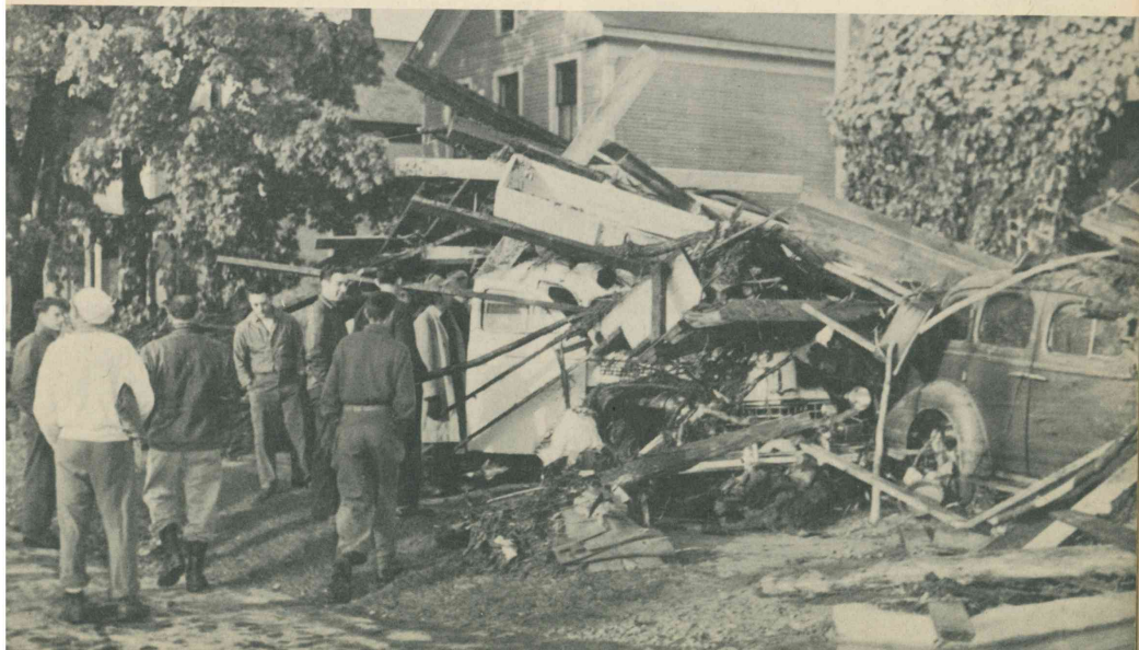
Two motor vehicles buried in debris
