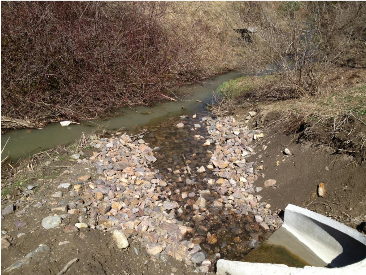
Clean water from a newly constructed stormwater treatment practice discharging into the turbid waters of Potash Brook.
