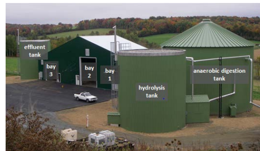
Figure 4: VT Tech Biodigester
