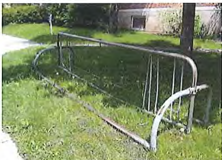
Broken Bicycle rack outside of the Bennington Public Library
