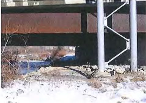
The trail will cross under this VT267 overpass.
