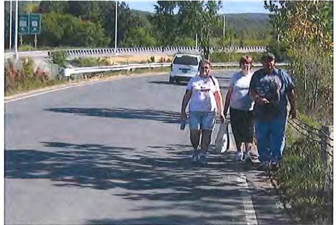
Applegate residents walking on Orchard Road. Guardrail and embankments force pedestrians to walk in the travel lane.
