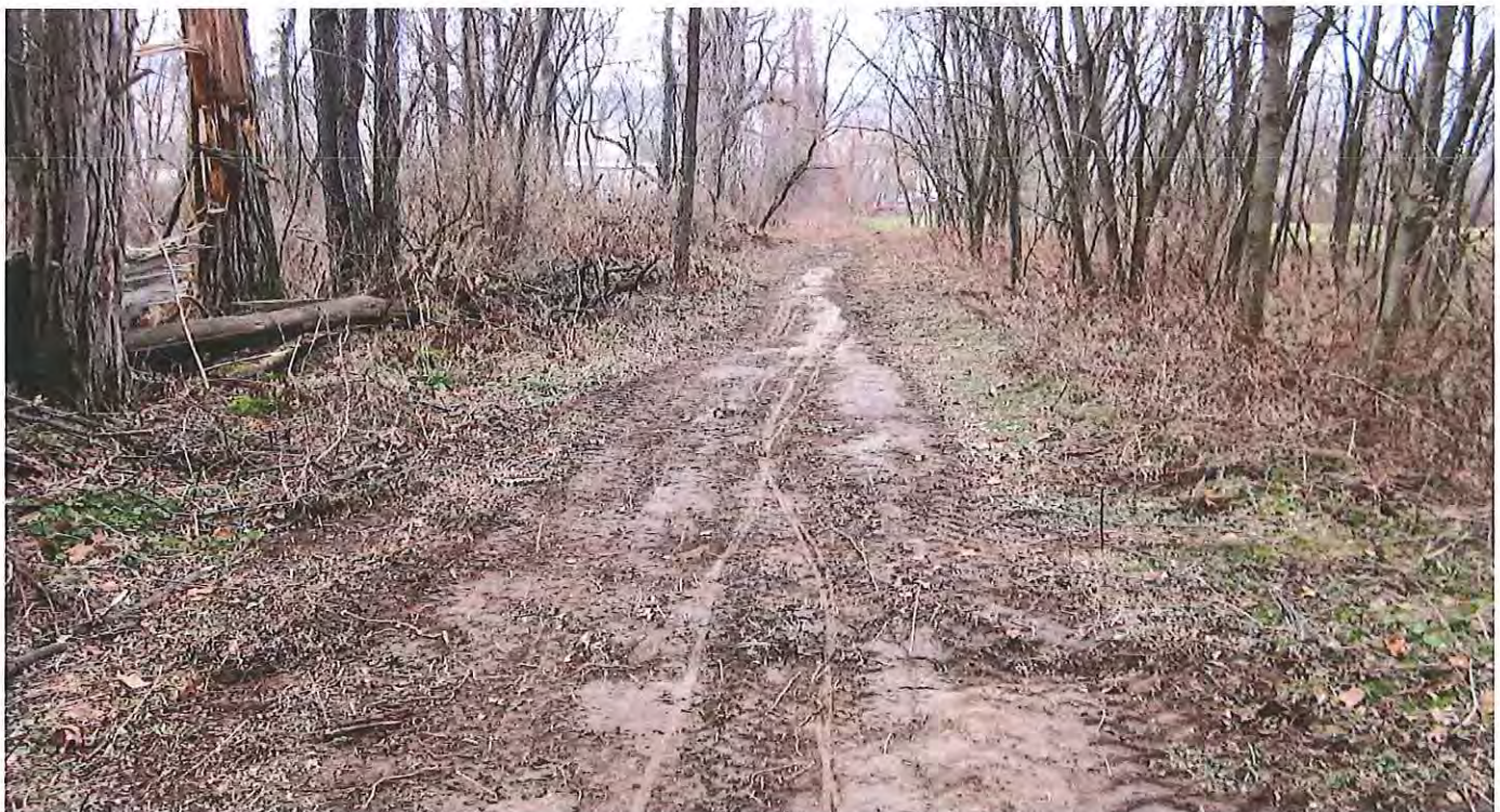
A cleared section of trail awaiting gravel.
