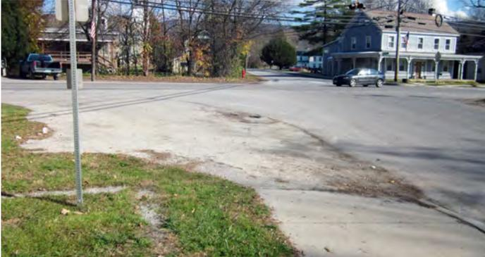
*The sidewalk and curb end before the intersection exposing pedestrians to fast, wide vehicle turns.*
