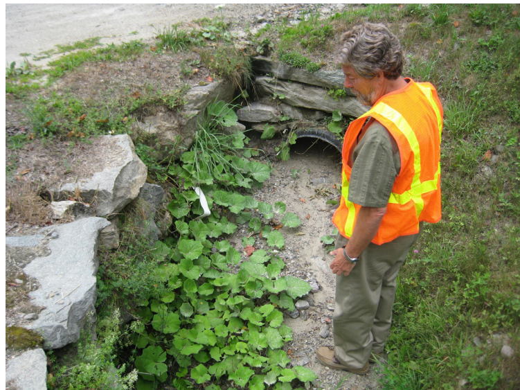
Program Director David Antone surveys a ditch in Landgrove that is full of sediment. With the help of VLR, the small town in Bennington County has made substantial improvements to its 15 miles of local roads.
