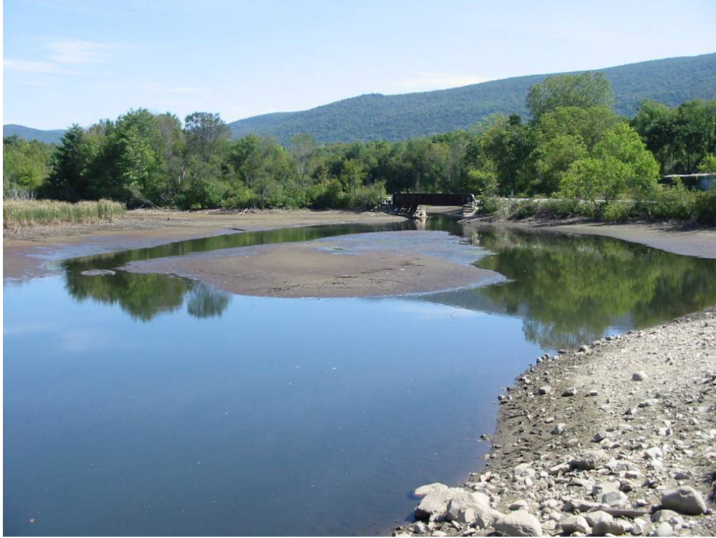
Figure 20: Dufresne Pond Dam. Photo of Dufresne Pond Dam impoundment after drainage (Roy Schiff, 2011)
