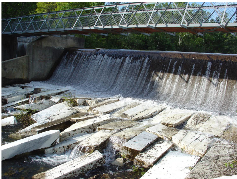
Figure 17: Dufresne Pond Dam, Photo courtesy of Roy Schiff, 2011
