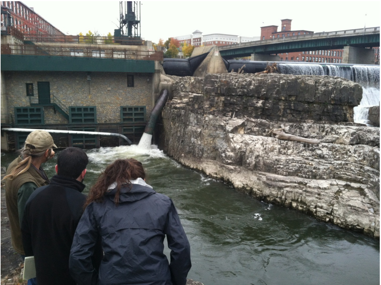
Figure 12: Winooski One Dam.
