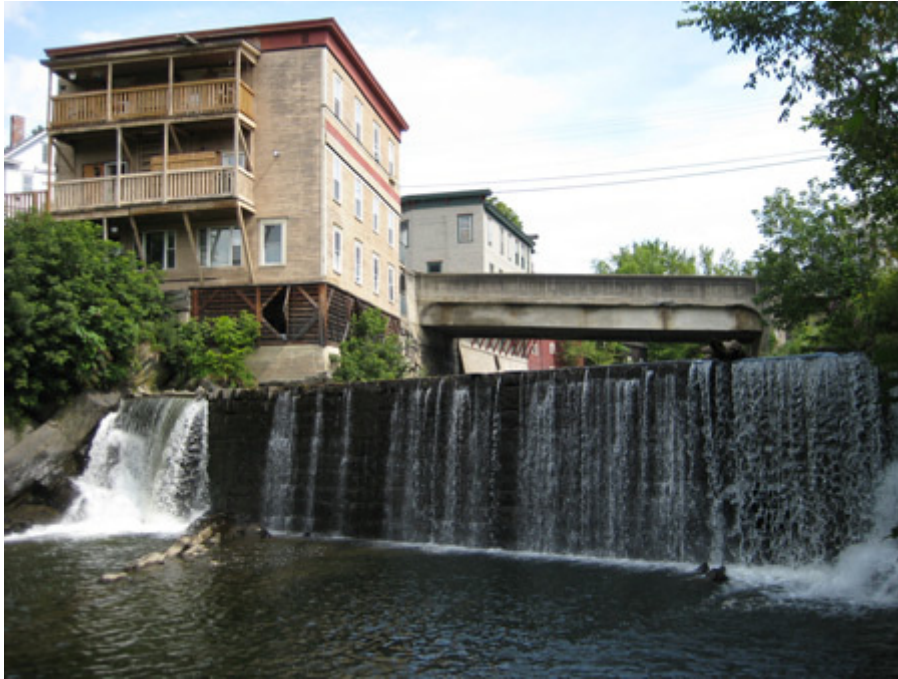
Figure 14: Batchelder Mill Dam. Photo from the Town of Plainfield website, http://www.plainfieldvt.us .
