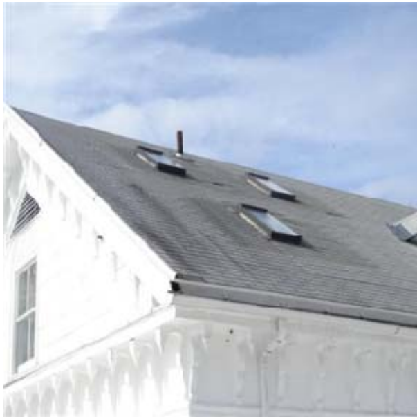
Wood cornice of original house
