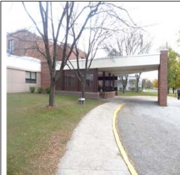
Main front entrance
