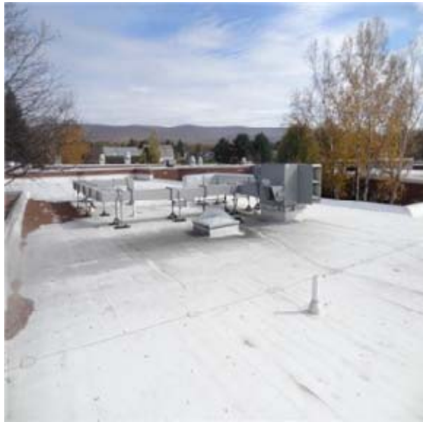
Main roof finishes
