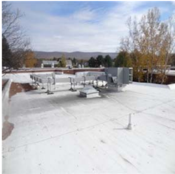
TPO roof membrane
