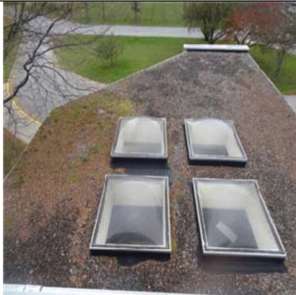
Flat roof over entrance
