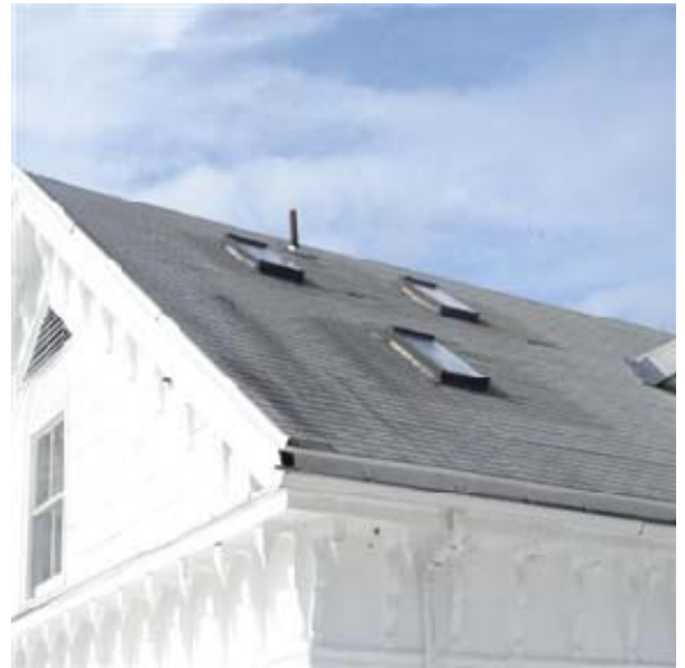
Asphalt shingle roof on original building
