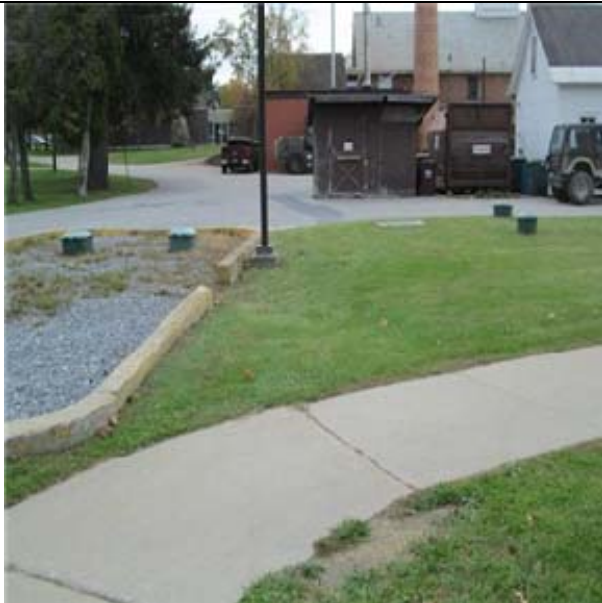
Underground propane storage tanks
