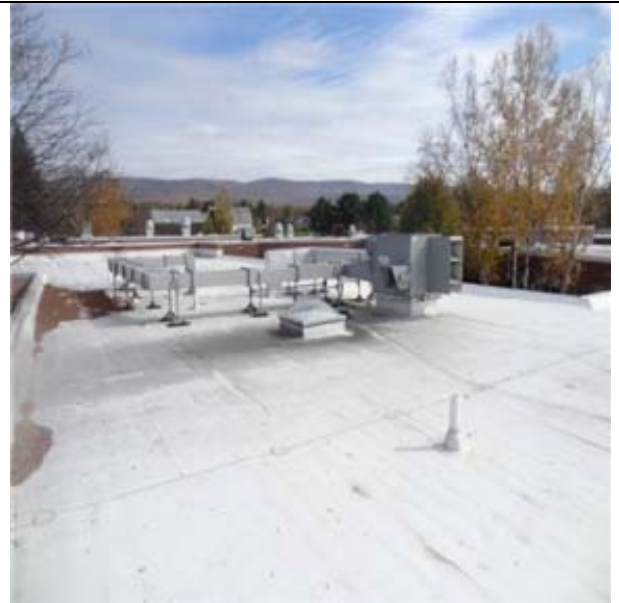
Main roof finishes
