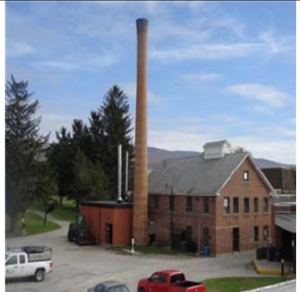
Asphalt shingle roof on old boiler building
