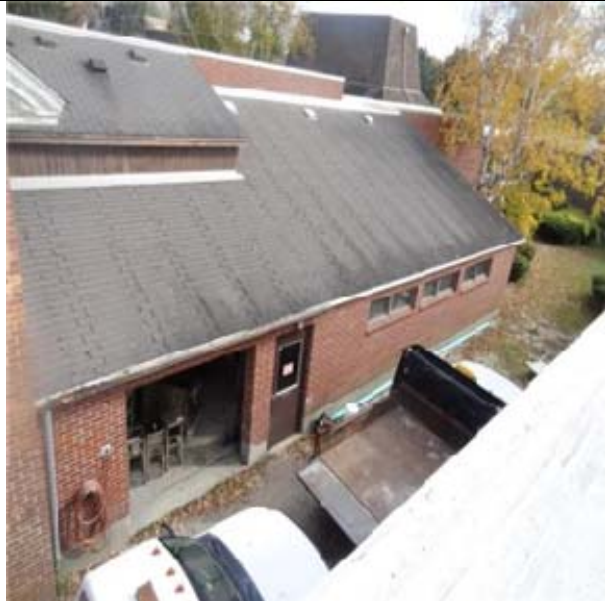
Old boiler and maintenance shingle roofs
