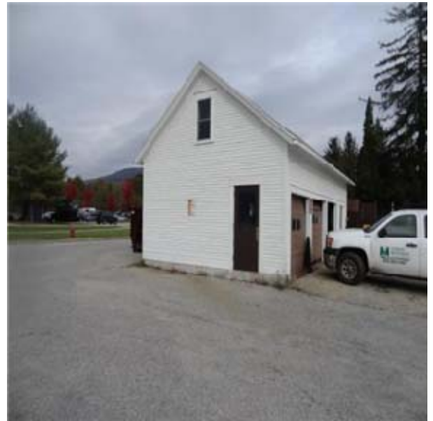
Garage wood siding
