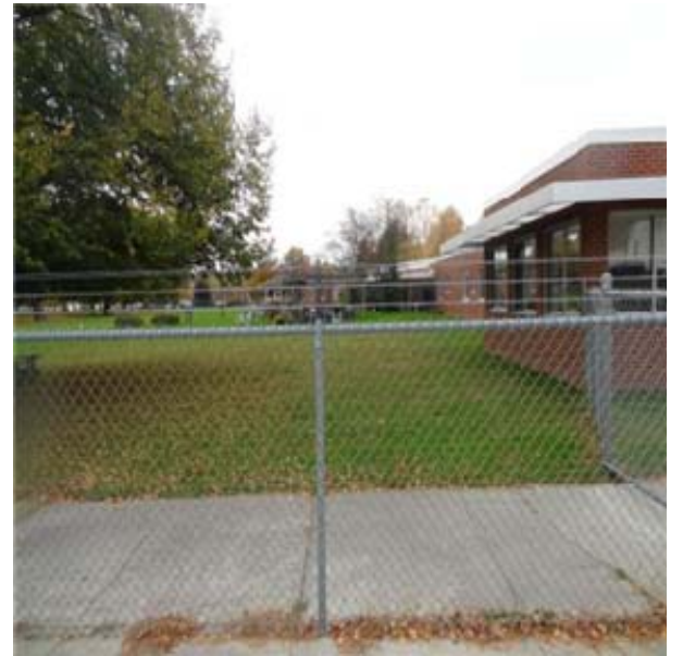
Security fence along Dementia Courtyard
