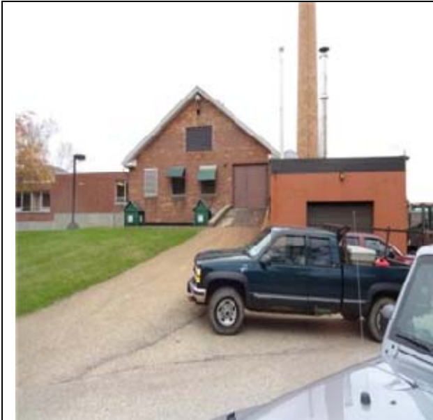
Old boiler laundry building
