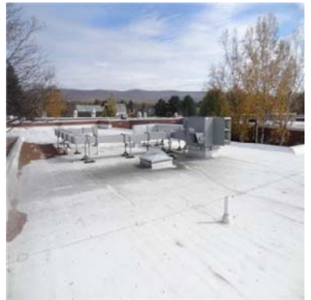
TPO roofing, North Wing
