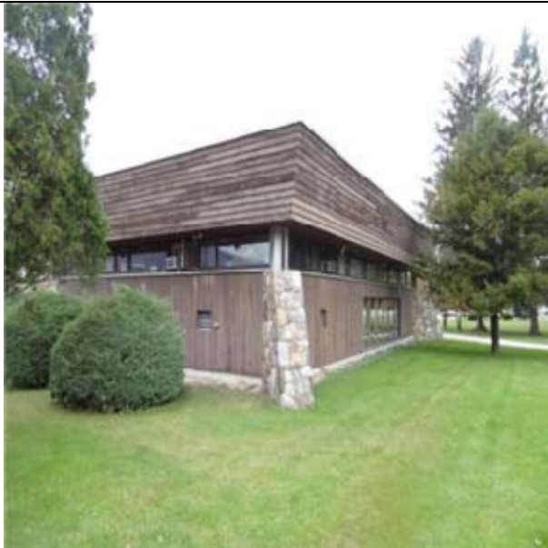
Vertical and horizontal wood siding
