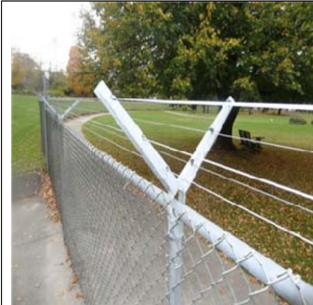
Security fence along Dementia Courtyard
