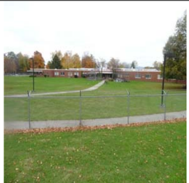
Security fence along Dementia Courtyard
