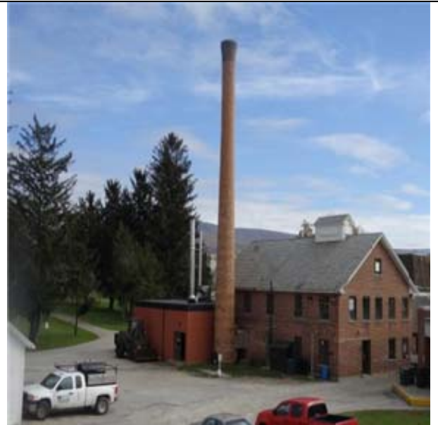
Old boiler and laundry
