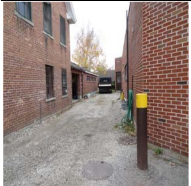
Asphalt pavement at Maintenance Service Drive
