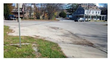
The sidewalk and curb end before the intersection exposing pedestrians to fast, wide vehicle turns.
