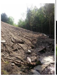
Figure 18. Before and two weeks after implementation: a bioengineering fix to a seriously eroding brook in Williston is taking hold. VYCC conducted the work. Photo credit: VTDEC
