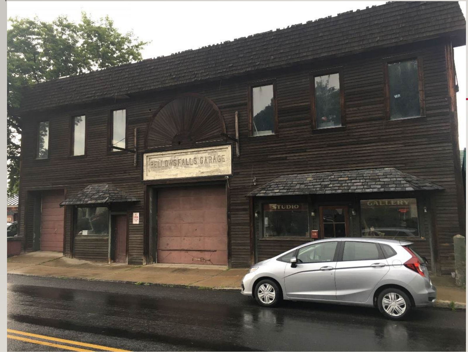
Front View from Rockingham Street
