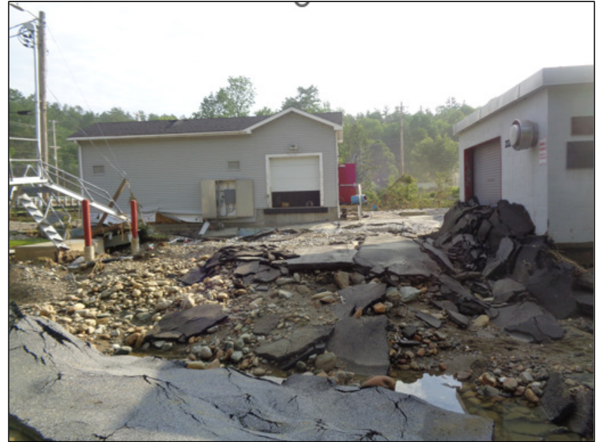
Headworks and control buildings
