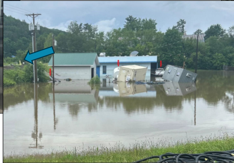
Flood Waters at Facility Buildings Slope to left is the lagoon
