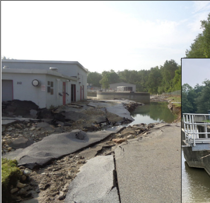
Entrance to Wastewater Treatment Facility
